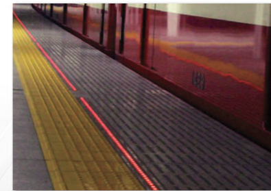
Thread Lines (Flash Light Strips along the Platform Edge) P8
