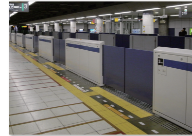
Partial-Height Platform Screen Door Systems P4-P6
