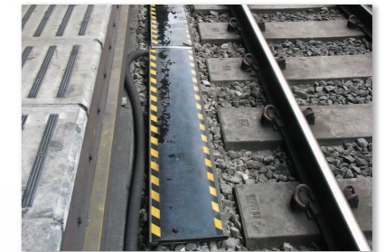
Passenger Falling Detectors (Mat Switches) P10
